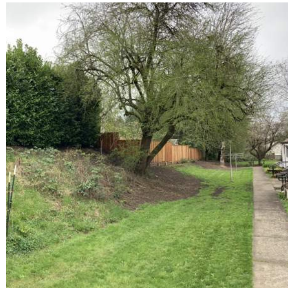
Southern Retaining Walls
